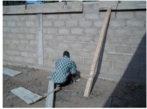
Construction of the wall
